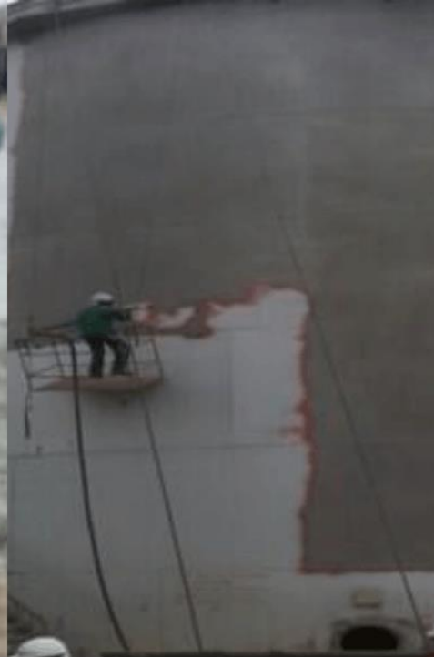
Tank and Other Mechanical Construction
