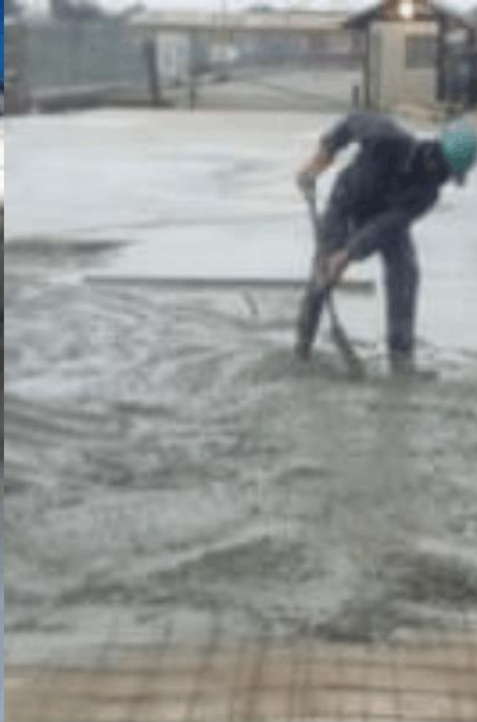
Road Works and Embankments
